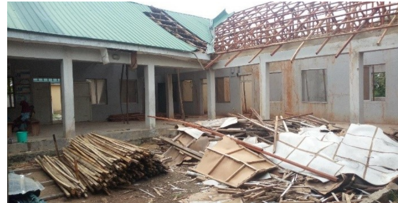
Construction Commence After FTM Intervention
