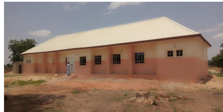
Kabo Hospital, Kano State
